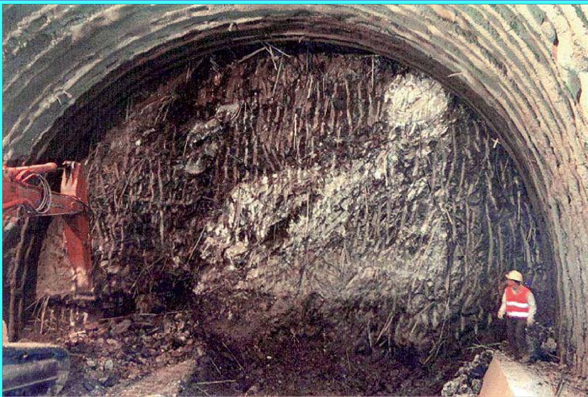
Colle Pece Tunnel. Face reinforced with fibre glass structural elements. Ground: scaly clays. Overburden: ~ 25 m [Lunardi Proyect]
