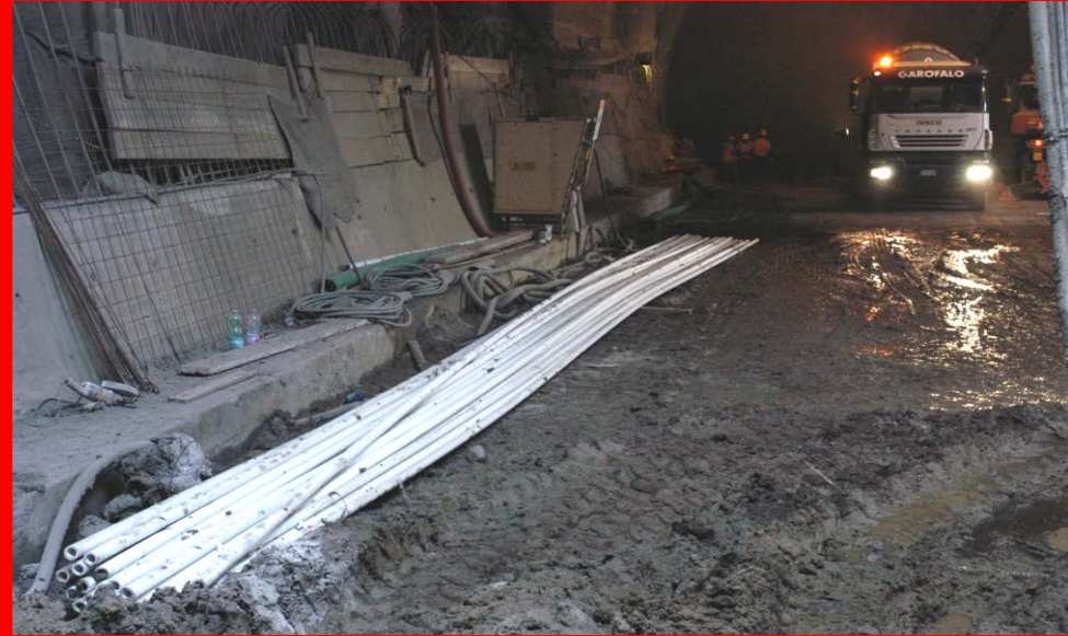
PHASE 2: Positioning pipes
