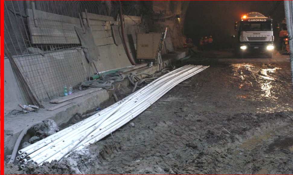
PHASE 2: Positioning pipes
