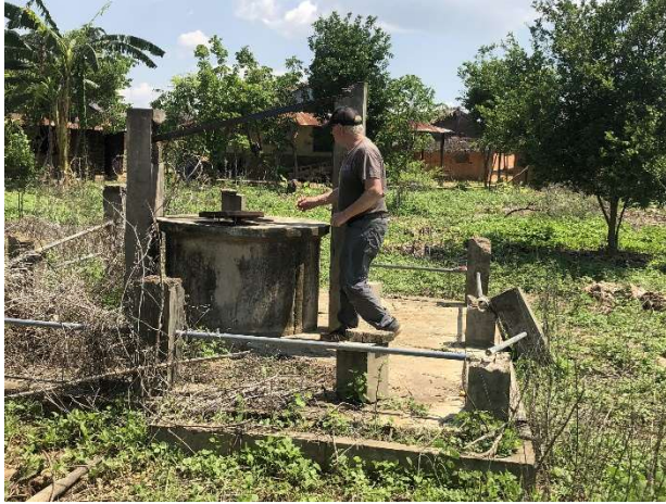
Pic. Abandoned bucket well at Ampihoara village
