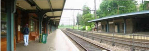
Existing Station Platforms
