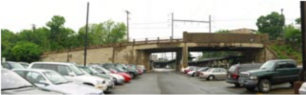
Existing Greenwood Avenue Bridge
