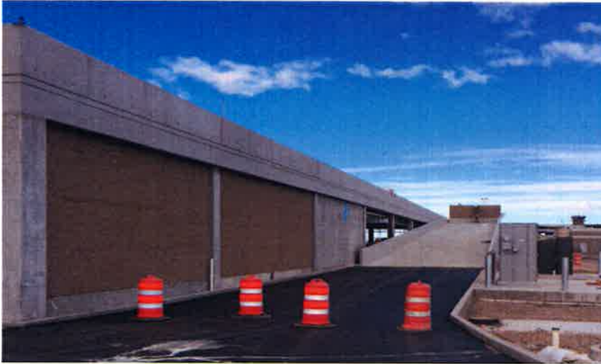
QTA East Ramp Completed and Approach Road Paved.
