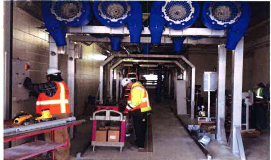
QTA Carwash Equipment Installation in the Westernmost Bay
