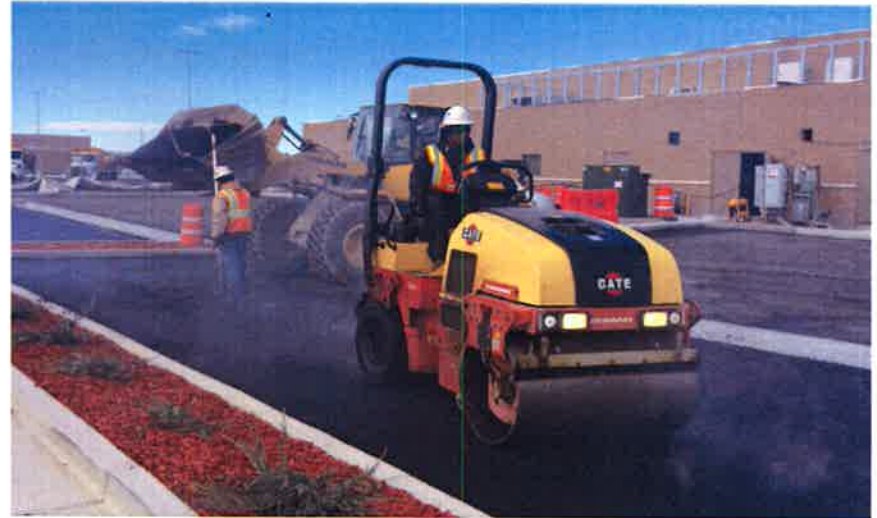
Asphalt Paving at RSS 'A' Parking Area.
