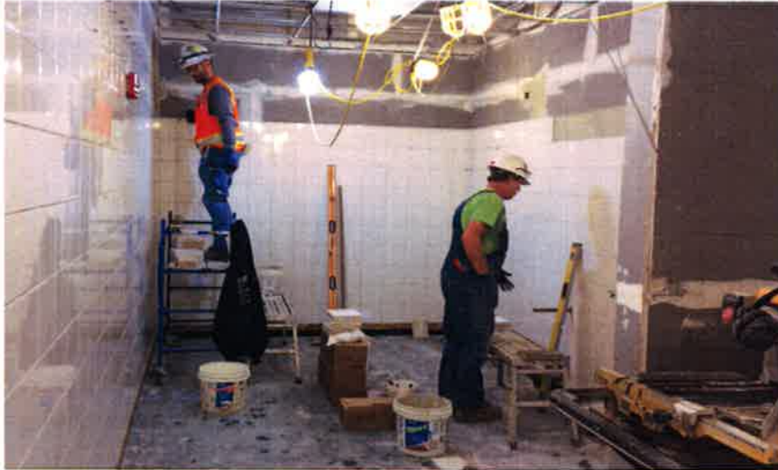
Installing Ceramic Tile in QTA West Locker Room/Restroom
