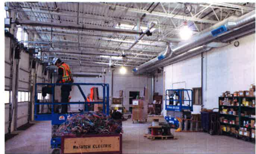
Work Bay Progress in RSS 'C'
