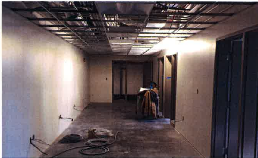
Interior Progress in RSS 'B' Admin Area
