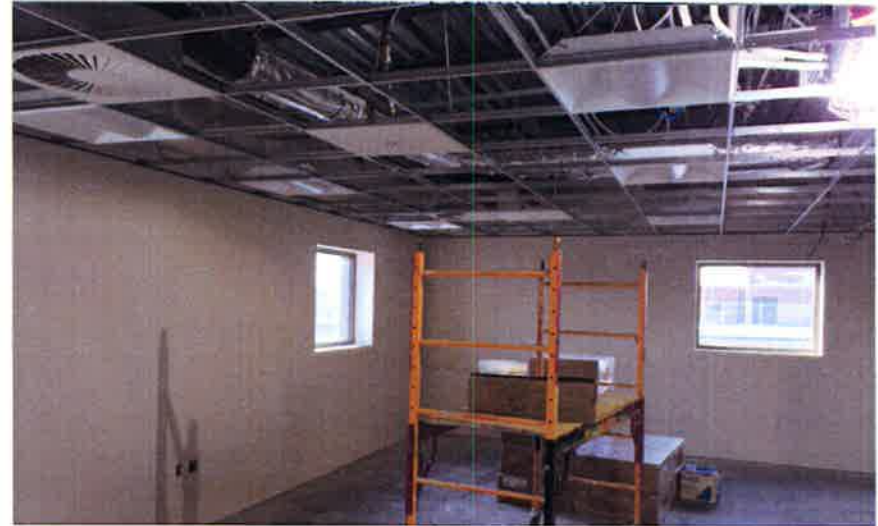
Interior Progress in RSS 'A' Admin Area
