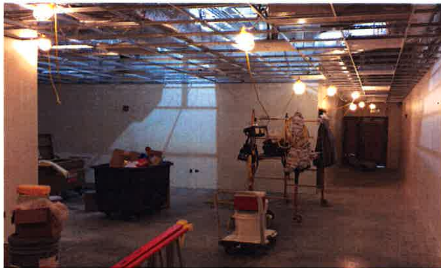
QTA Admin Build-out, HVAC Ducts & Returns, and Lighting
