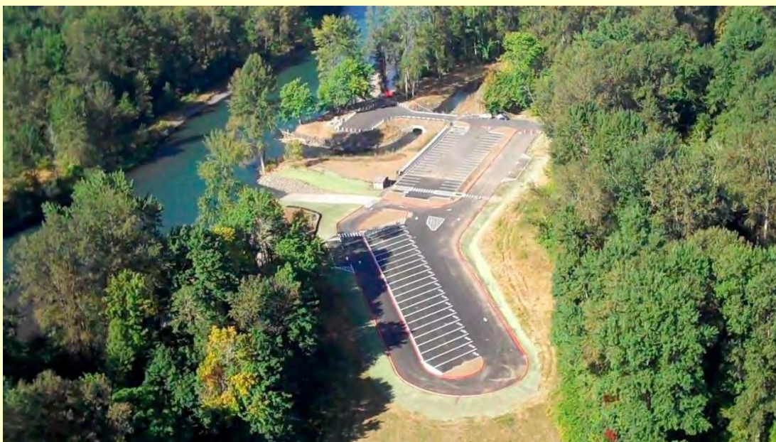
The newly constructed Mill Race intake, parking area, and boat launch (Source: RaptorViews, 2012)
