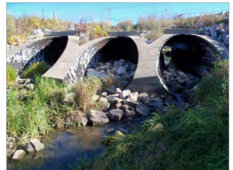
Photo 9: The downstream inverts of Structure 61 (three parallel pipes) sit at least twelve inches above the water surface.
