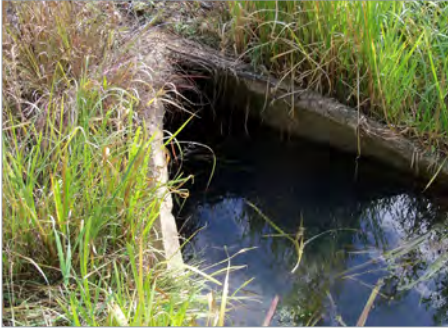
Photo 1: The end section edges of Structure 19 are spalling and are exposing the rebar reinforcement.
