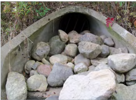
Photo 4: The channel end section of Structure 31 is approximately half-full of riprap.
