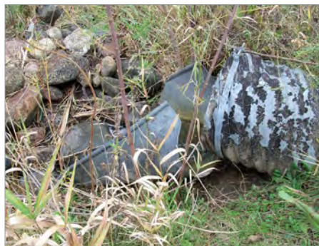
Photo 5: The channel end section of Structure 45 is detached from the pipe.
