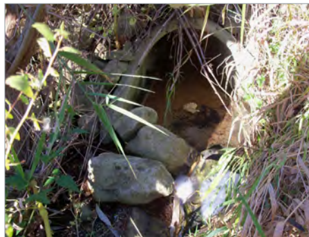
Photo 8: Suds were observed at the channel outfall of Structure 52 indicating a possible illicit discharge.
