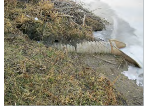
Photo 3: Gully erosion has formed around the west end of Structure 29 from the shoreline to approximately ten feet landward over the top of the pipe.
