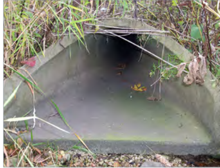
Photo 2: The as-built plan for Structure 41 shows that a trash rack was installed; however, no trash rack is present.
