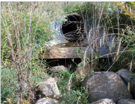
Photo 7: The end section of Structure 94 is undermined by approximately twelve inches.
