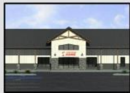
Hankinson's Post Hardware Hank was destroyed in a fire in fall 2019. Owners Jill and Jeremy Post are planning to open their new 10,000 square foot hardware store in April 2020.
