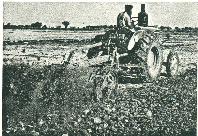
Tilth control demonstrated—by using the shield. Greater variation still can be obtained with 'Selectatilt'. ('H' trailing Rotavator on the same field—West Pakistan).
