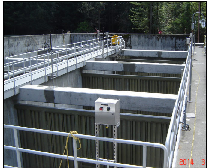
“Vertical” installation of Fiberglass baffle walls Installed at Russian River, CA
