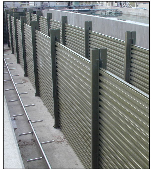
Typical Baffle Wall Installation Keegan’s Bayou Houston, TX
