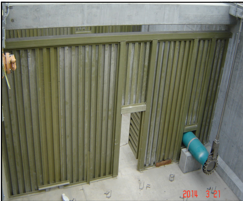
Basin Installation at Russian River, CA
