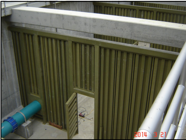
“Vertical” installation of Fiberglass baffle walls Installed at Russian River, CA
