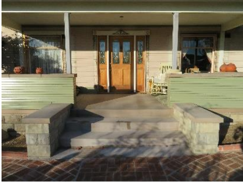
The rock face block gets placed on either side of the front steps (above) and flanks the finished porch steps (below). It's a close match to the original Hanawalt block foundation
