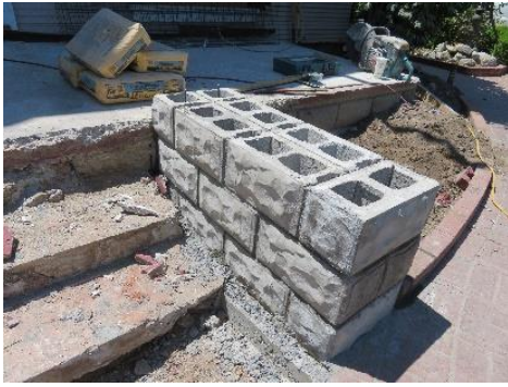
The rock face block gets placed on either side of the front steps (above) and flanks the finished porch steps (below). It's a close match to the original Hanawalt block foundation
