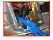
With the retaining rings removed, you can now slide the closing shim up and off the valve stem. If the shim gets "stuck" at the top of the valve stem, it is an indication the valve stem has mushroomed a bit. Some emery cloth/sandpaper is needed to remove the wide part at the top of the valve
