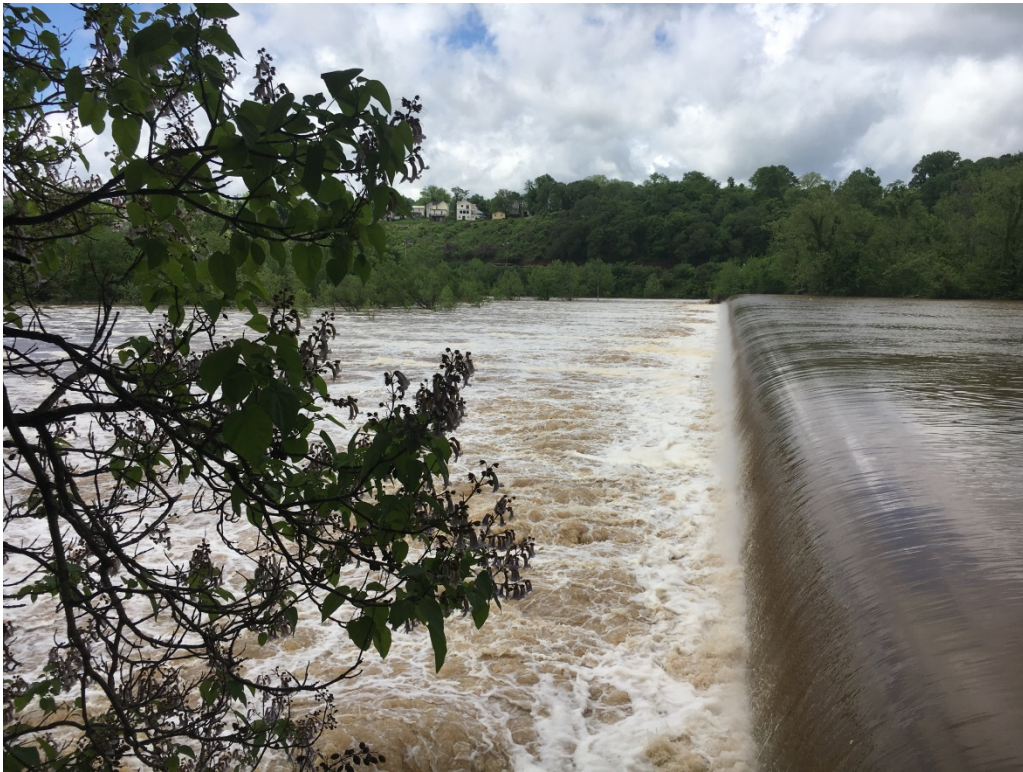
Photo 10 – Scott's mill Dam May 5, 2017 – High Flow about 25,000 cfs
