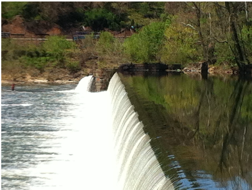
Photo 7 – Scott’s Mill Dam April 2016 – 1,800 cfs
