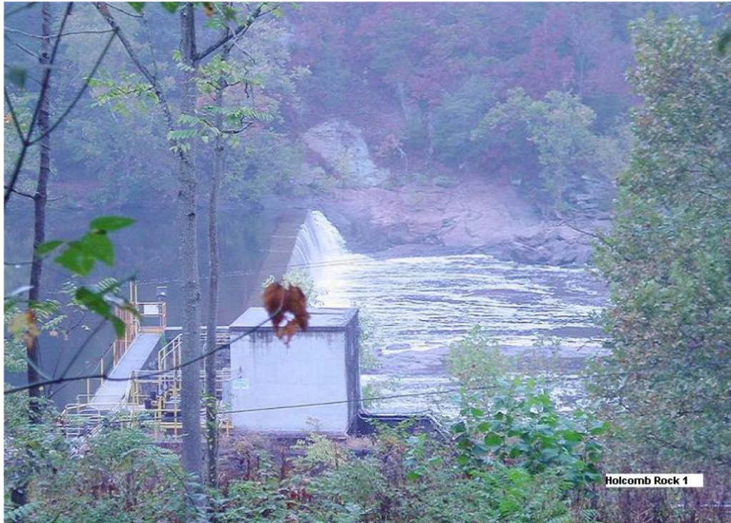
Photo 5 – Holcomb Rock Dam
