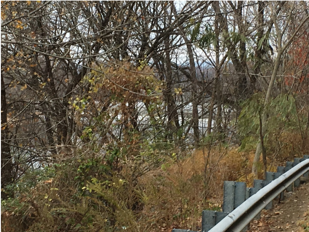
Photo 18 – November 28, 2016 Scott’s mill Dam from River Road in Defoliated Season
