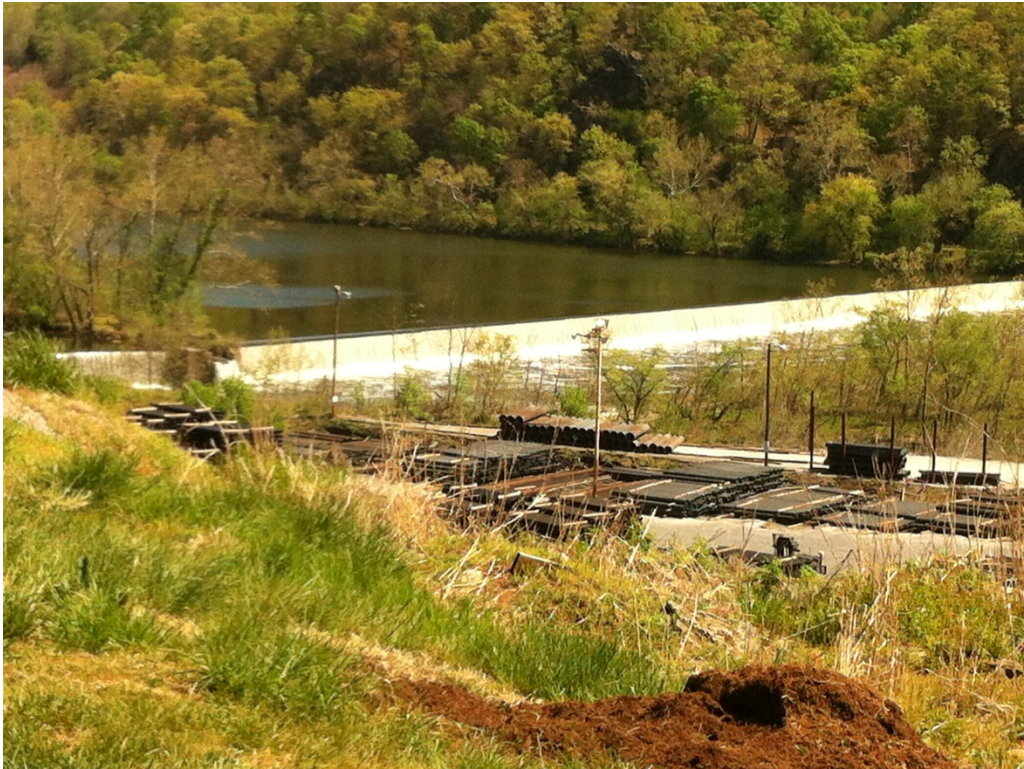
Photo 20 – April 20, 2016 Scott's Mill dam Viewed from North Side of Norwood Street (Note Pipe Storage Area)
