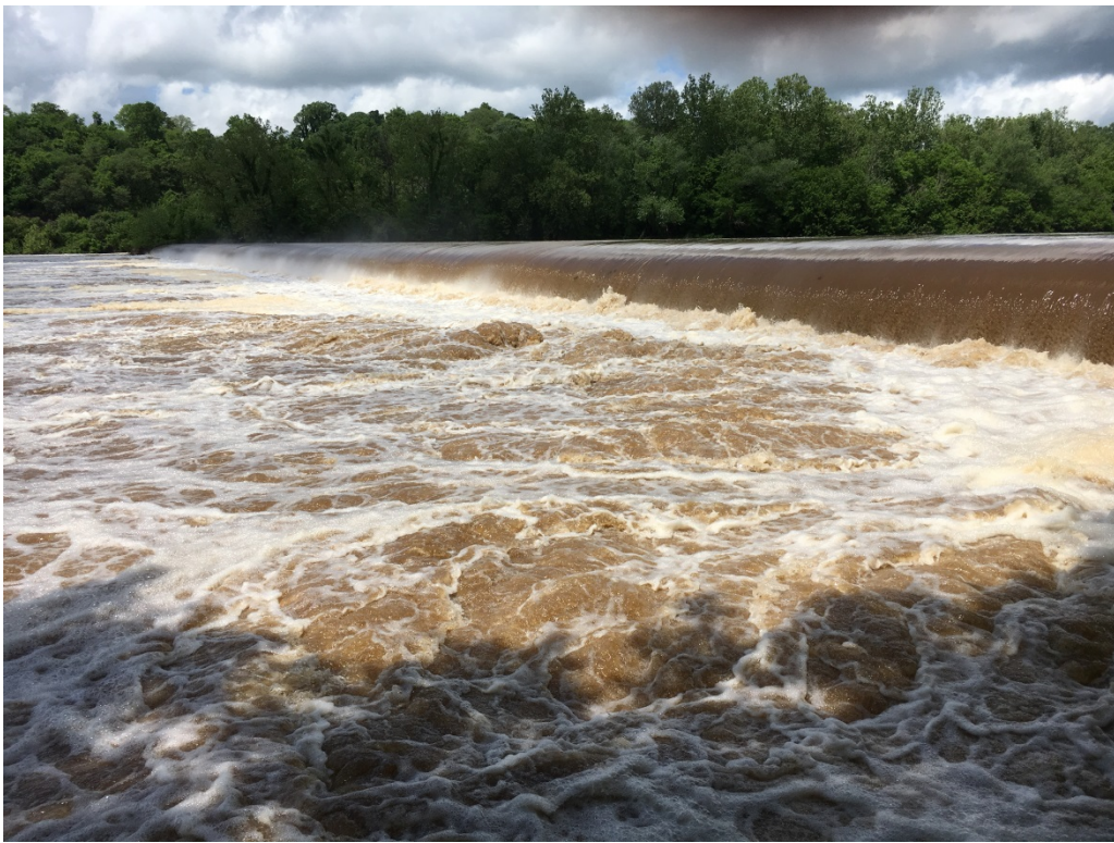
Photo 11 – Scott’s Mill Dam May 5, 2017 – Note Turbulent Flow and Reduced Head
