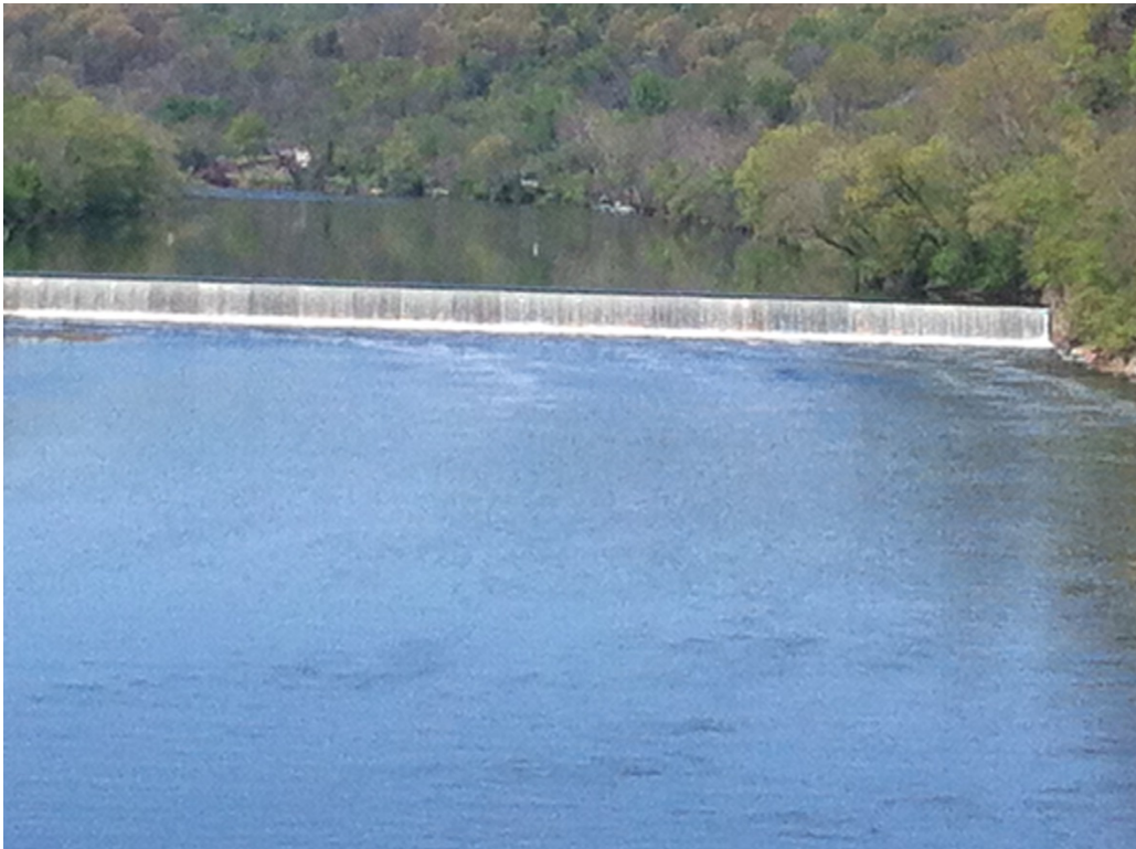
Photo 19 – April 18, 2016 Scott’s Mill Dam as viewed from 5 th Street Bridge
