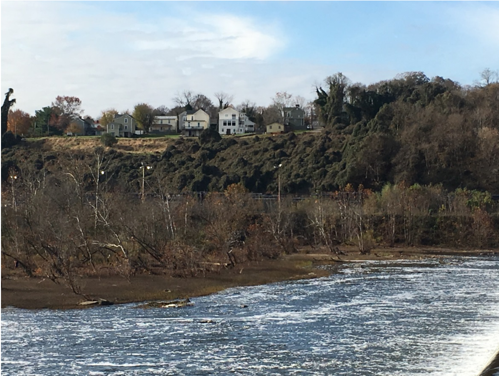
Photo 22 – November 14, 2017 Views of Homes on Norwood Street with Views of Scott's Mill Dam (Note Downstream Island in Foreground)
