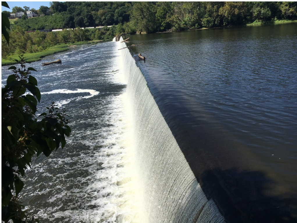
Photo 8 – Scott’s Mill Dam September 12, 2016 – Low Flow about 800 cfs
