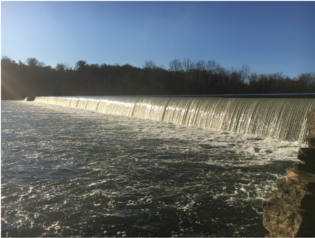
Photo 13 – Scott’s Mill Dam February 2, 2017 – Average Flow 3,200 cfs
