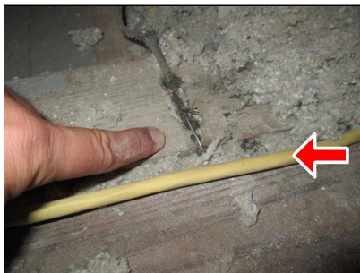
B. Item 8(Picture) bare wiring near attic access
