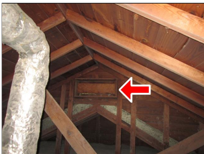
D. Item 3(Picture) sealed gable vent
