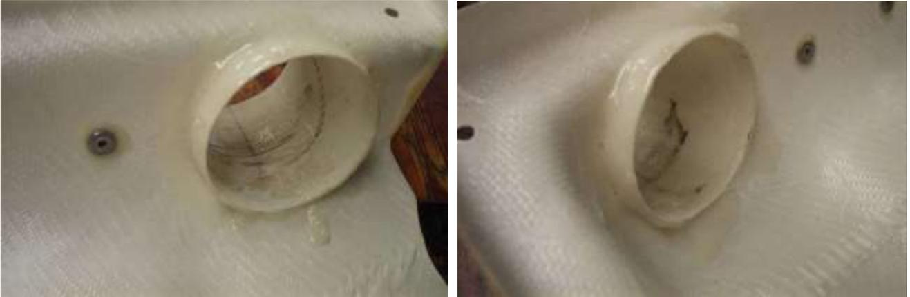
**Figure 34. Air Filter Box Plumbing – Incorrect**
