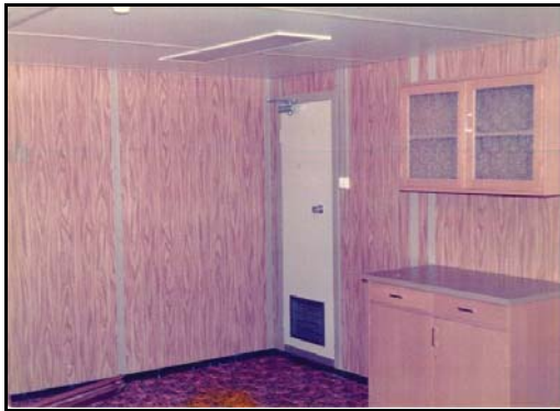
Fire doors and bulkheads
