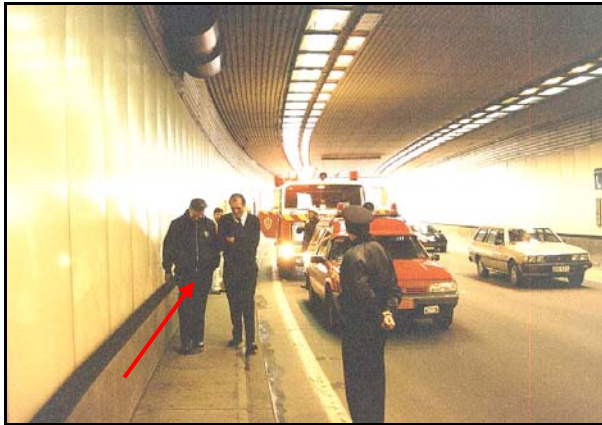
Barry Eadie in the Kings Cross tunnel during detector testing for false alarms.
