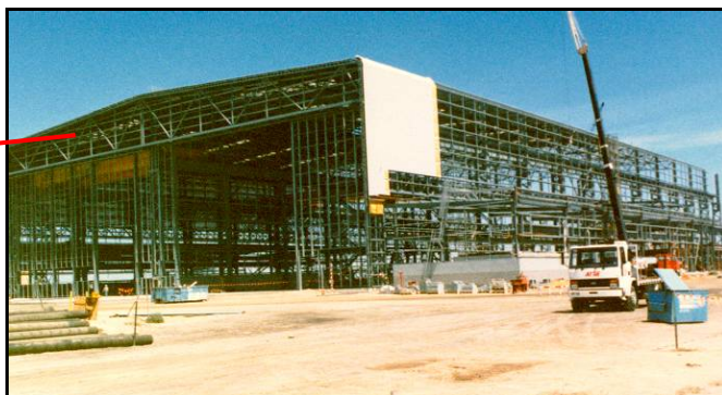
The ASC Hull and fit-out building
