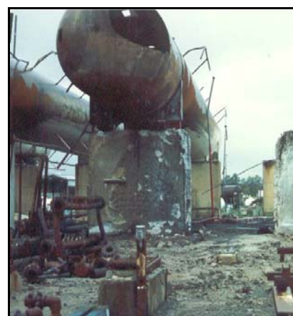
The destroyed Boral facility
