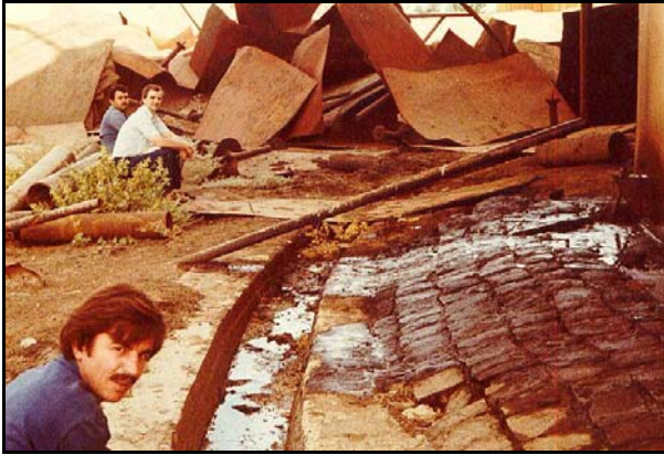
Ken Stewart in background next to an oil tank that had caught fire – killing five workers
