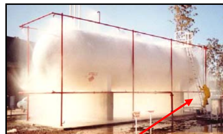
AMCOR plant – me checking system
