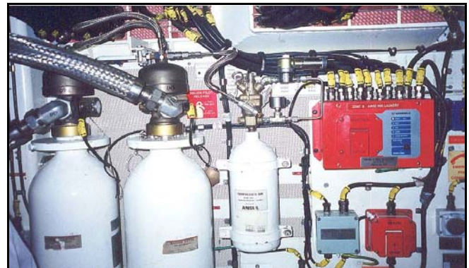
A fire system in a Collins Class submarine
