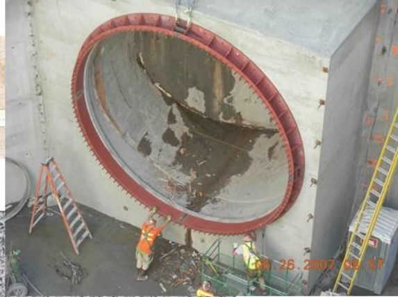
A 20 ft Entry Ring with Inflatable Seal at 80ft deep
