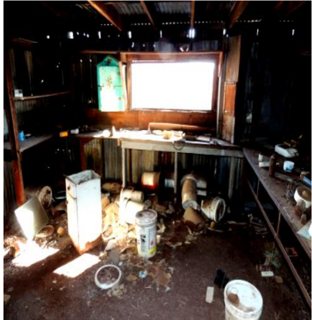
Inside one of the rooms in the building above.
