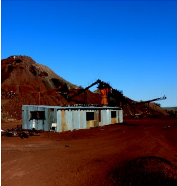
One of the old abandoned buildings at the Cinder Mine
