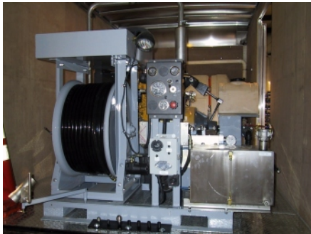
Skid Mounted Van Installation
