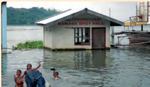
Health facilities under water following Typhoon Ketsana.
