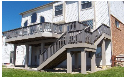
New, safe, reconstructed deck
