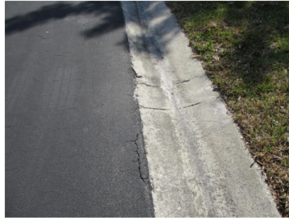
Minor gutter deterioration and cracks
