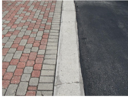
Cracks at pavement edge
