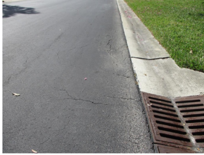
Pavement cracks
