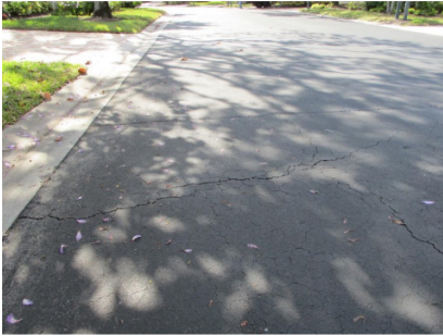
Pavement cracks
