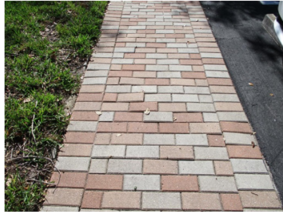
Displaced pavers at entry sidewalk
