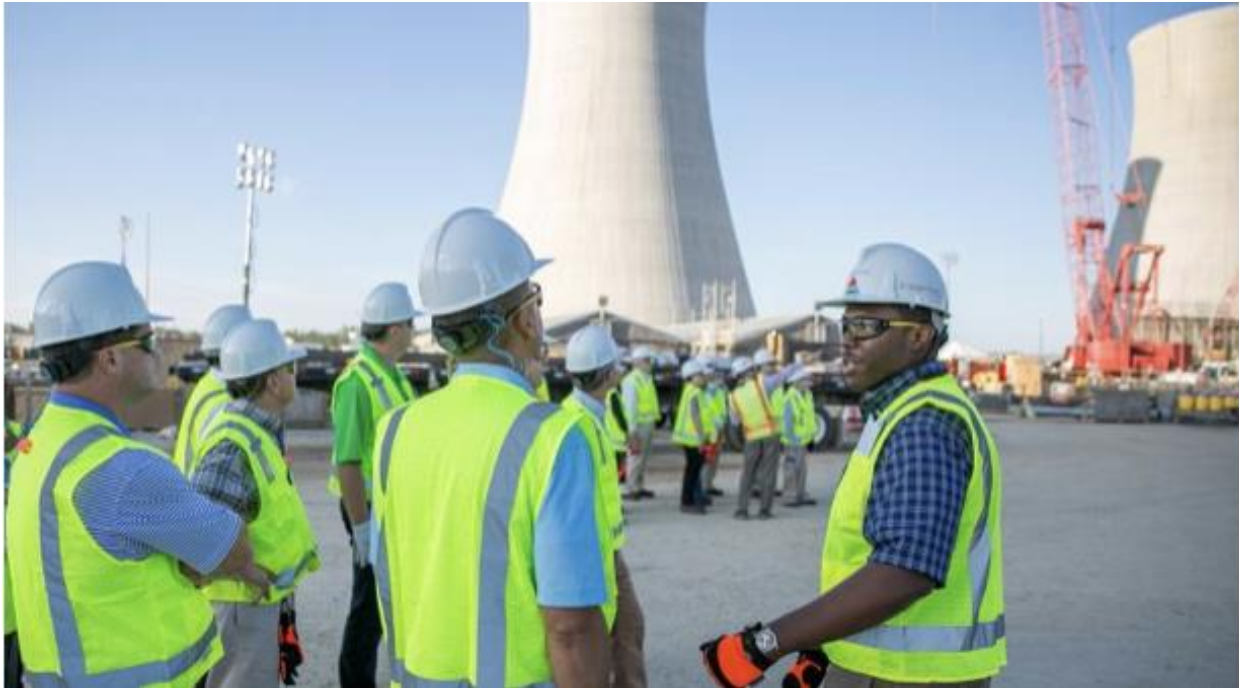
Southern Company considers giving public tours of the Vogtle 3 and 4 nuclear plant construction site essential for explaining the benefits, importance and progress of the project. (Image: Georgia Power)
