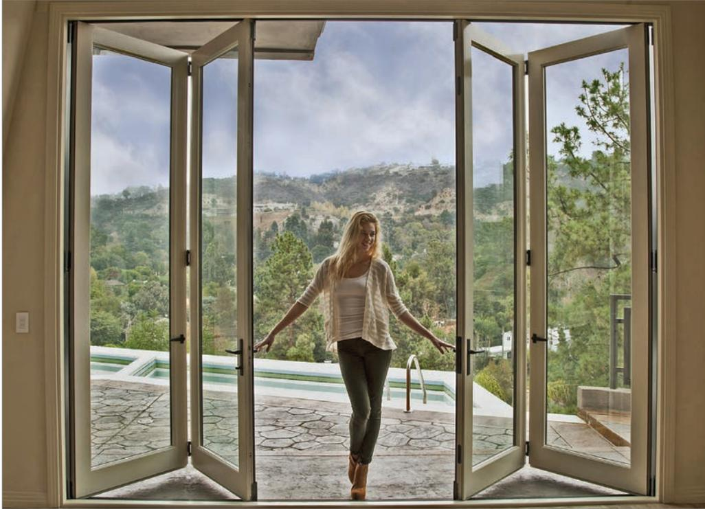
and hinged together to slide accordion-style and stack against one edge of the opening or the other.
