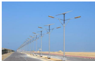
Solar PV LED Street Lighting
