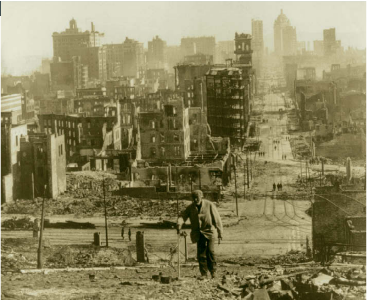
A city levelled Fire damage, above, and, inset, houses close to collapse after the 1906 San Francisco earthquake
