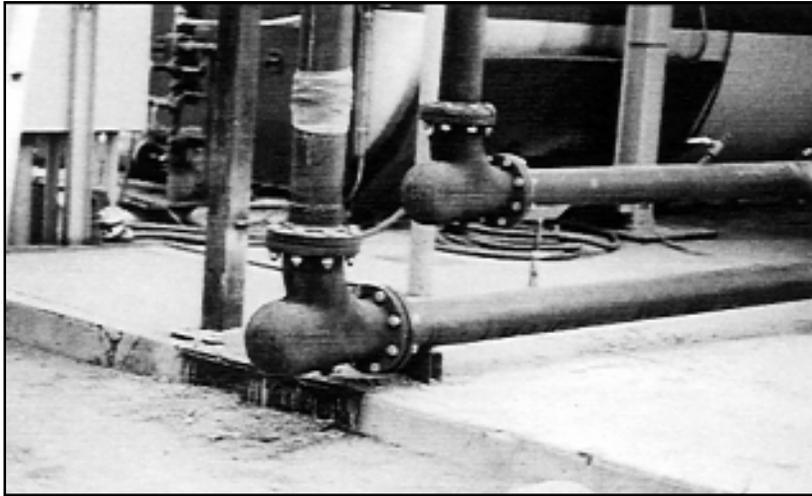
*Smart Elbow™ ends elbow wear problem in paving plant.*
