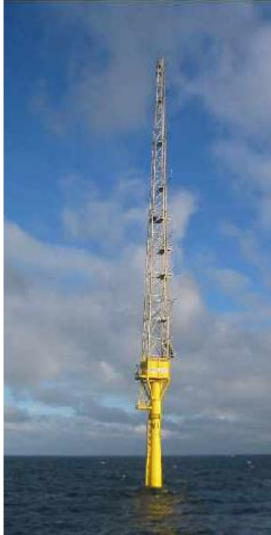
Figure 4: The met mast mounted on the completed monopile
