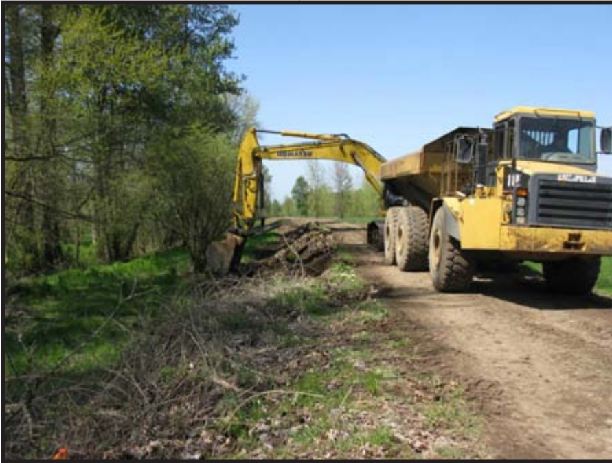
2009 levee removal project
