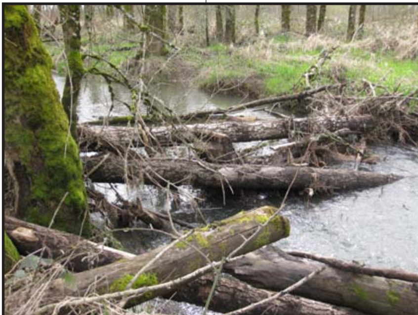
Large woody debris placed in Willamette River side channel at Green Island in 2008
