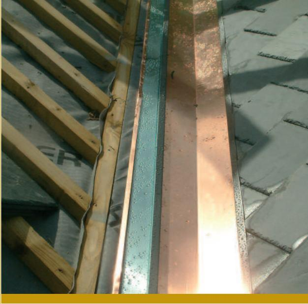
**Valley linings:** are another popular product coming in 2 linear metre lengths with an interlocking detail and factory made top intersection that simply click into place. A highly attractive feature compared to traditional lead linings. We manufacture to suite all sizes and pitches.
