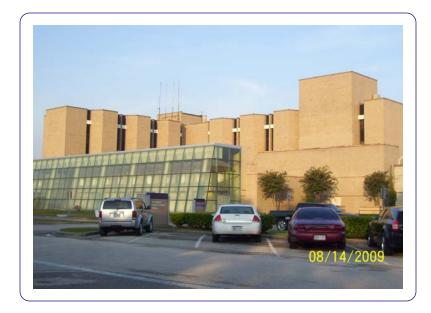
The subject hospital building is a multi-story hospital comprised of a two tower buildings and several adjoining lower roof areas. MHHS retained the services of PCI to prepare specifications and drawings for replacement of the roof on the Southeast Tower. The building is an 8-story steel-framed structure with brick masonry veneer and strip windows constructed in the early 1970s.
