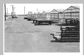
Low cost, plastic film greenhouses at the Ahrens range in Osseo. The houses were used for bedding plant production. Wide, paved driveways permitted loading plants on trailers or trucks directly from doors or openings in the sidewalls of the greenhouses. (Photo by author)
