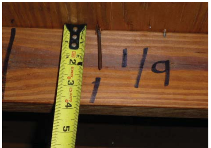
#3 ROOF DECK ATTACHMENT 8d NAILS
