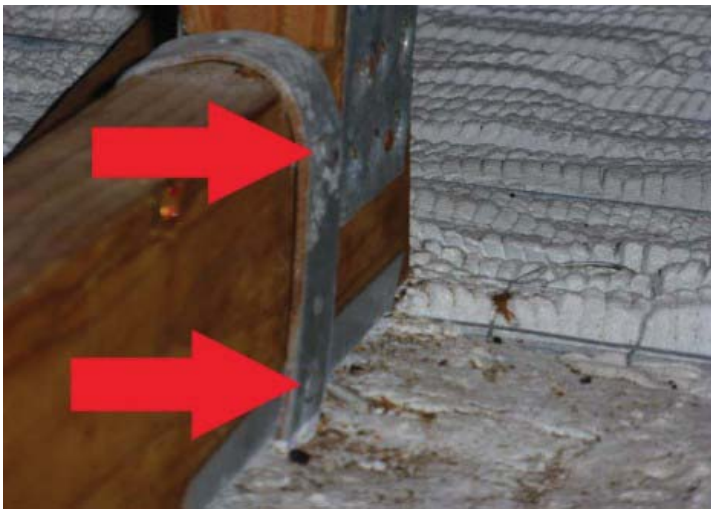
#4 ROOF TO WALL ATTACHMENT FACE SIDE
