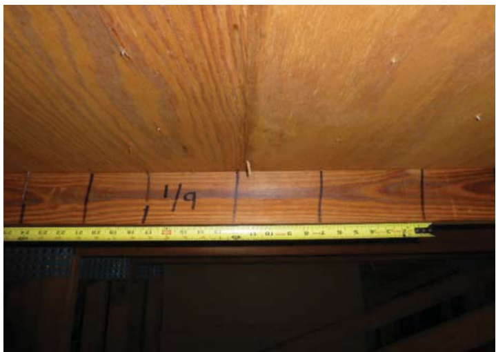
#3 ROOF DECK ATTACHMENT 6" X 6" NAIL SPACING
