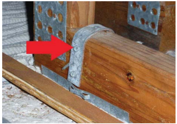
#4 ROOF TO WALL ATTACHMENT OPPOSITE SIDE
