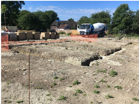
Excavating and concreting foundations.
