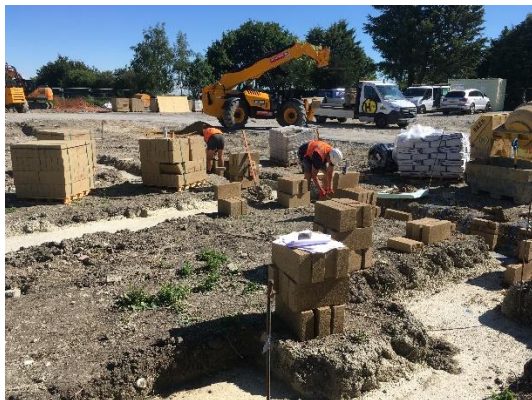
Block work below DPC started Monday 15 th June.
