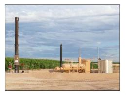
In the past, with oil storage tanks in place, oil was processed through "combination" vessels like the one pictured here. These are horizontal heater treaters with vertical separators built in, and they are traditional in Colorado. Often these horizontal vessels (green arrow) are fitted with pre-heat tubes to heat the incoming well fluids. Once heated
