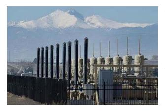
As population increases and spreads out, it inevitably gets closer and closer to legacy oilfield operations like those in this picture with the Rocky Mountains in the background. The vertical thin pipes on the lighter colored vertical vessels in this picture represent vent lines that carbon-based pollutants into the
