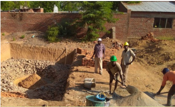
A hole for septic tank water disposal. We are using evaporation as well as percolation into the clay soil.. Two 10ft diameter towers double as distribution points and our back-up in case of system overload needing pump out...
