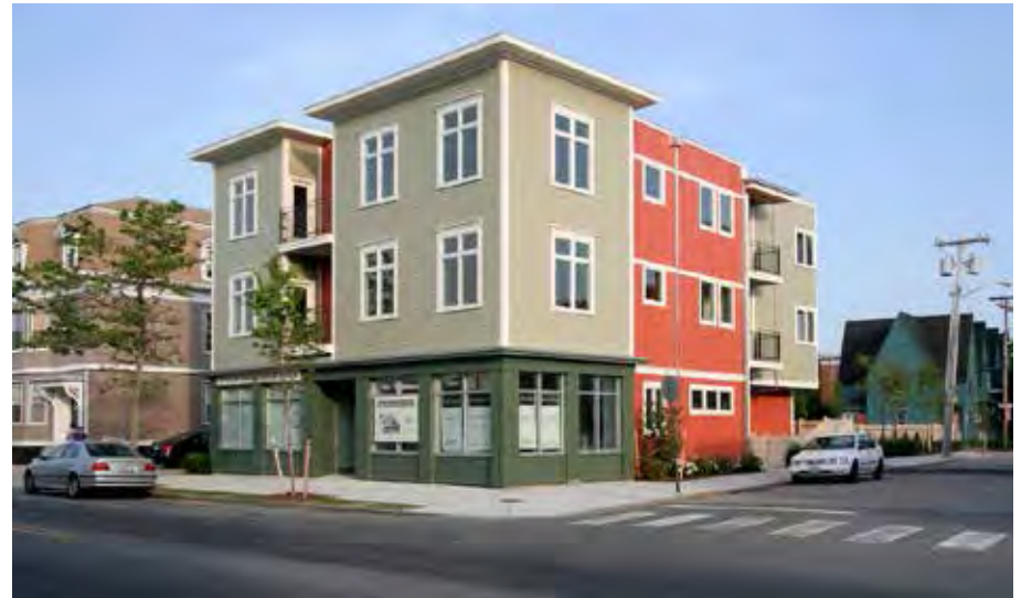
Improved connectivity between the rail stop and Airline Highway can provide additional opportunities for medium density mixed use projects as transit-oriented development.
