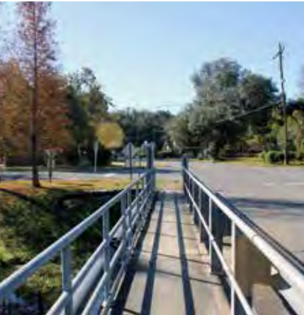
Existing pedestrian facilities
