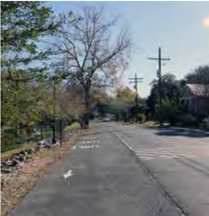
Existing bike facilities on W. Main Street
