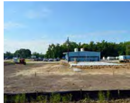
Construction along LA 44
