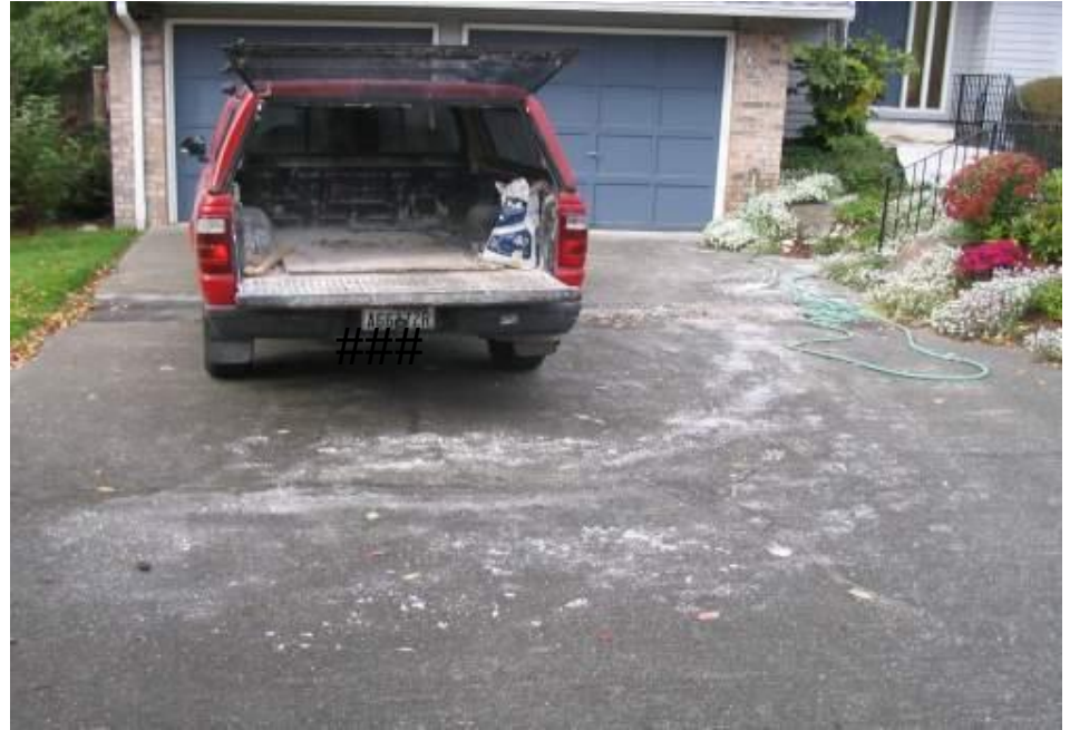
Uncontrolled popcorn ceiling removal job
