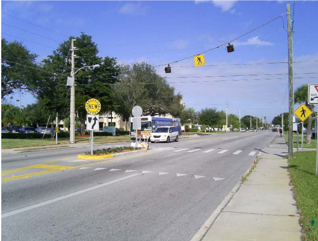
Figure 4. Photo. Northbound view of standard overhead beacon system and crosswalk at 58th Street N with advance yield markings.
