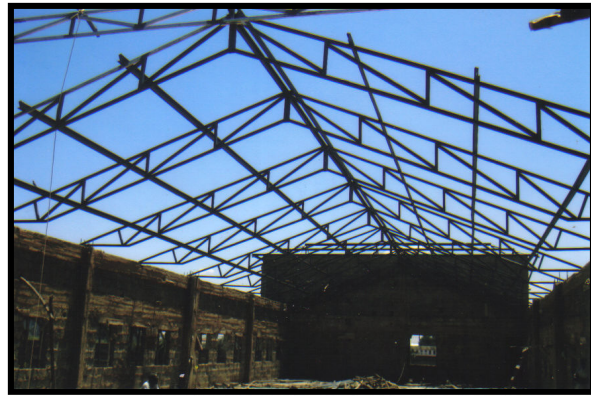
Third floor and roof under construction of the kitchen-dining hall building at the new Donora Campus, MCDC.
