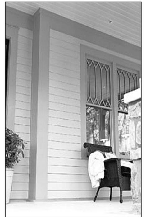
*As pretty as wood but better behaved, fiber-cement siding has become a favorite of architects, homeowners and builders. High resistance to fire, rot and insect damage, paired with excellent manners for paint retention and low maintenance, explain the appeal.* photo: courtesy of James Hardie Building Products
