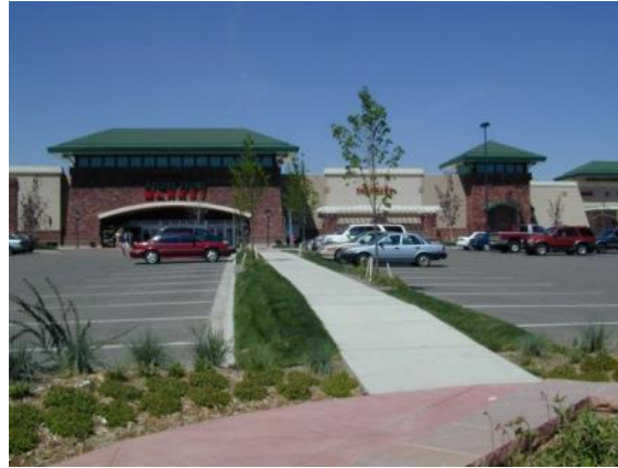
Figure 1218-E: This photograph illustrates how a sidewalk connecting the public sidewalk to the business can be integrated into the required landscaping.
