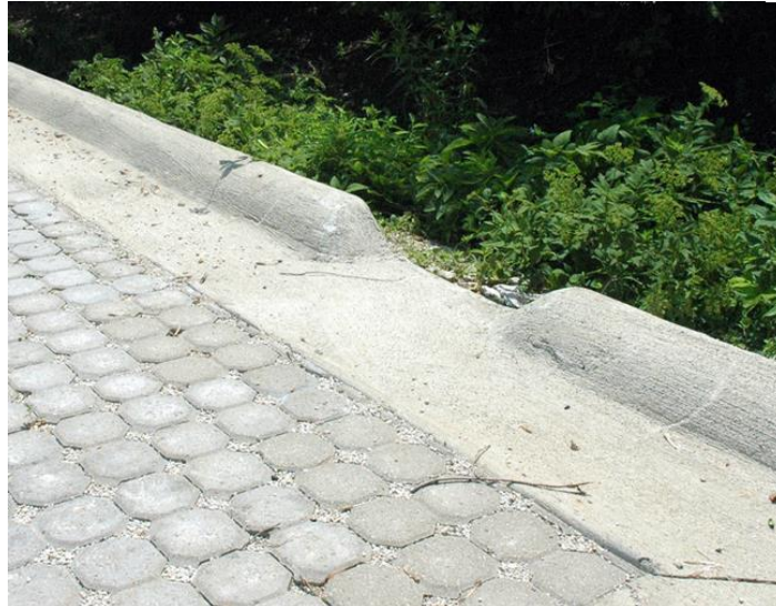
Figure 1218-C: Cuts in the continuous curb allow for stormwater to be directed into landscaped areas.
