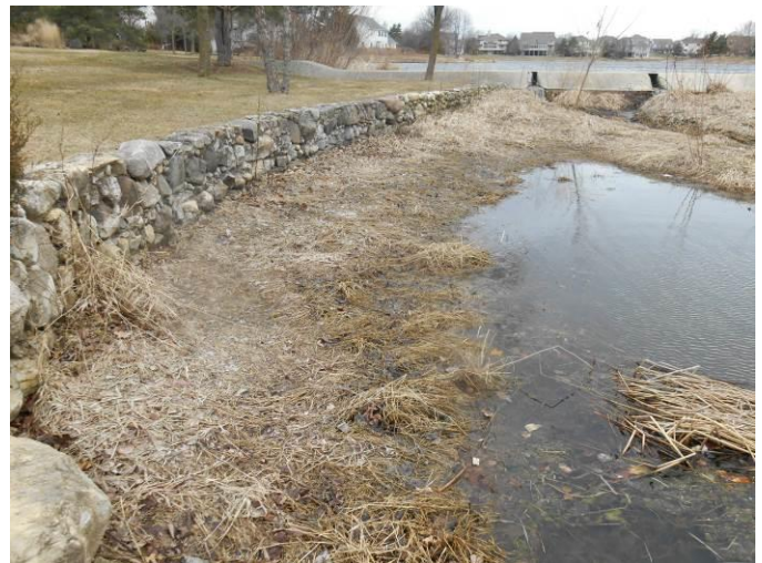
Overview of upper portion of spillway channel/stream with stone masonry retaining walls.
