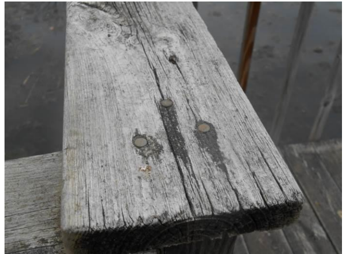
Large wood pier deterioration.
