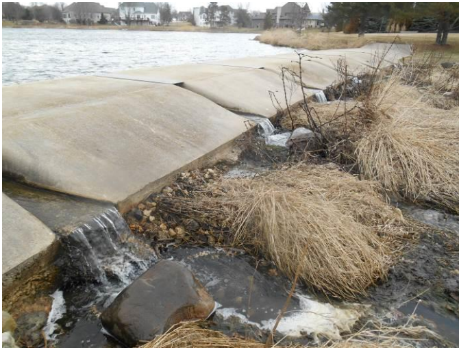
Spillway channels and buffers.
