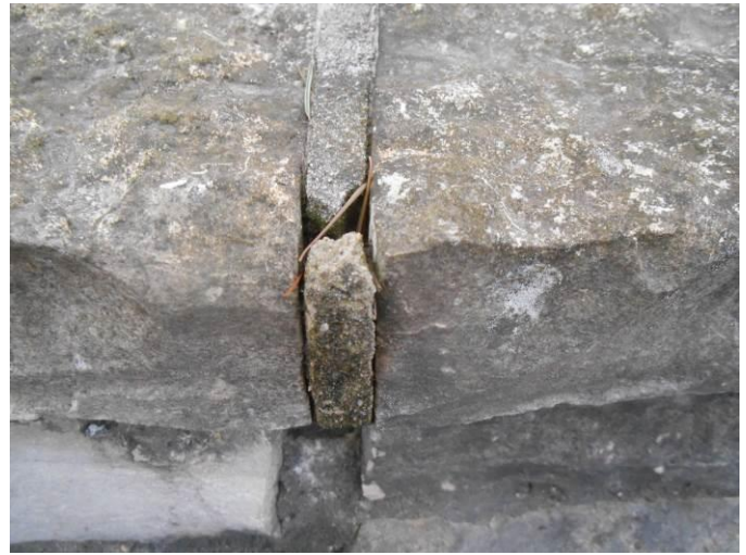
Deteriorated mortar and cracks allow moisture to penetrate leading to further deterioration. The entrance monuments require tuckpointing.
