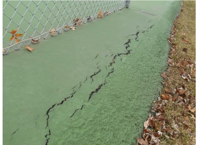
Minor cracking at north tennis court.
