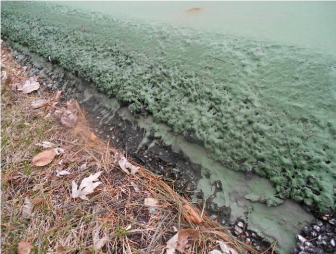
Tennis court asphalt overlay.
