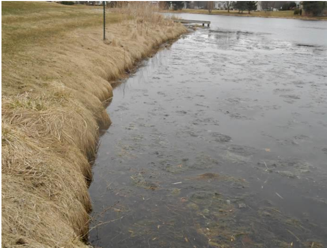
South east shoreline toe erosion.
