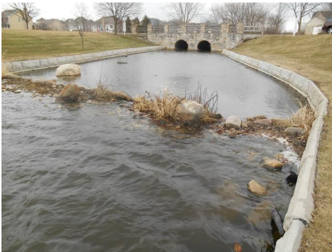
Overview of lower portion of spillway channel/stream with buffers and concrete retaining walls.
