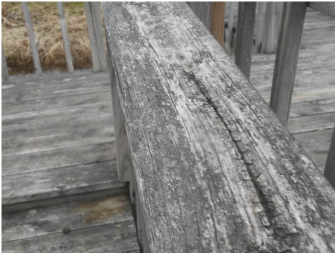
Large wood pier deterioration.
