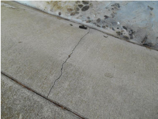
Minor cracking was observed in the spillway concrete. It is recommended that the cracks be sealed to limit damage that may occur due to moisture penetration and freeze/thaw cycles.
