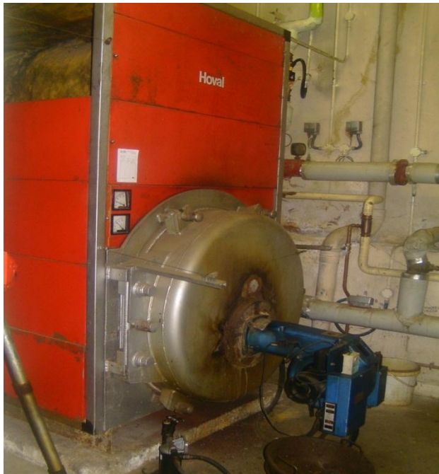
Current Pipe Work for Oil Fired Boiler
