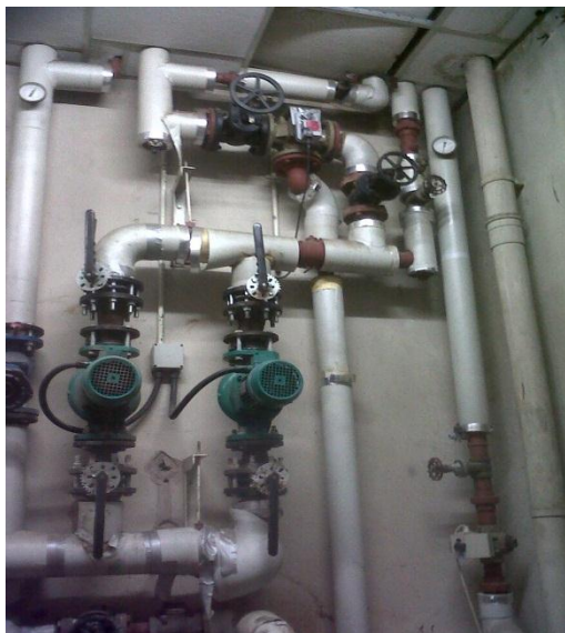
Current Pipe Work for Oil Fired Boiler
