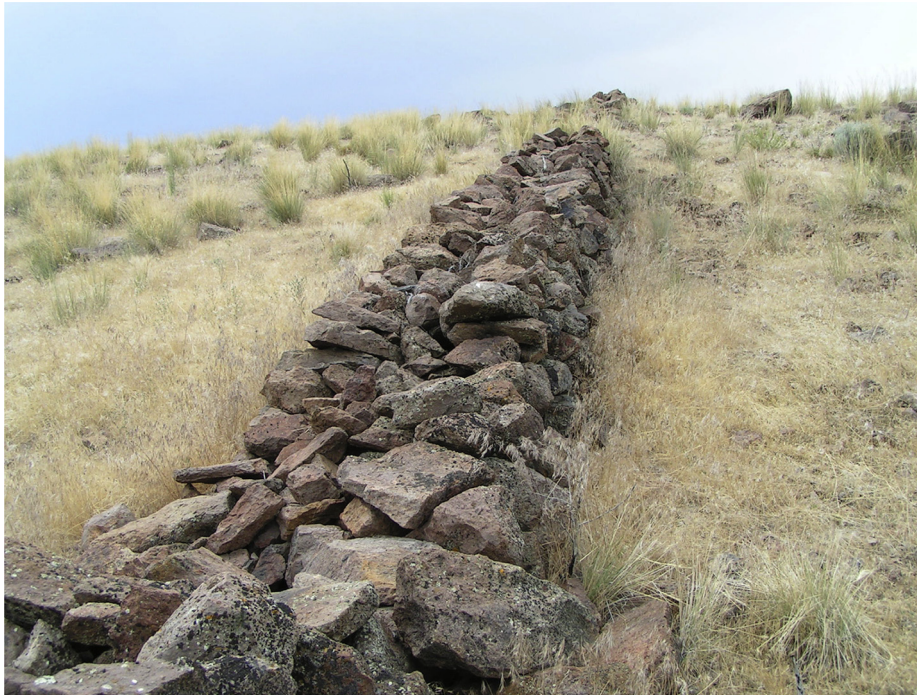
Fig. 2. A section of the Fort Sage Drift Fence, western Nevada.
