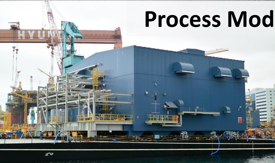
Loading Injection Compressor Module in Korea
