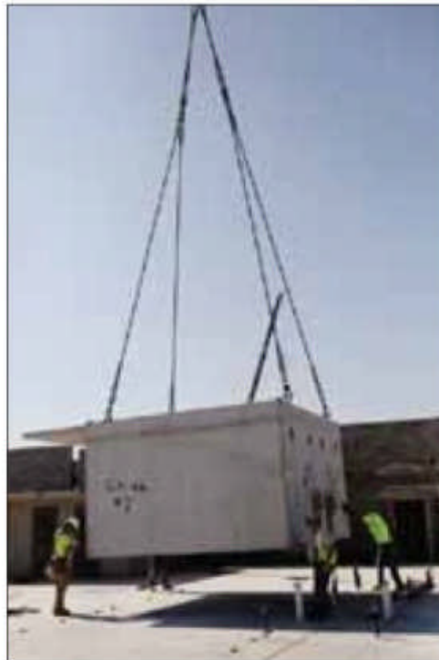
Above: A view of a two-person cell at the new Reno County jail. The site will contain 200 cells. Left: Workers place a cell at the construction site Wednesday. Below: An overall view of the jail construction and cell installation.
