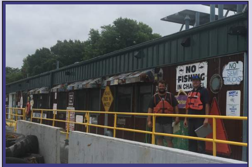
pictured above: Pat and Steve after repairing one of the AC units on the Classroom Barge
