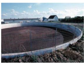
structure. The structure's purpose is to safely contain the manure and keep nutrient loss and pollution of downstream water bodies to a minimum by preventing runoff.
