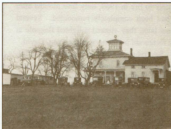
Pumps on left; Large building on right was later the Restaurant.
